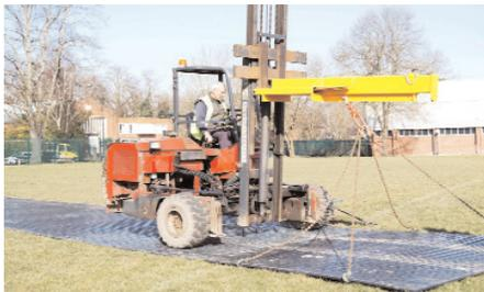
Regularly sweep away any loose earth or mud and, if necessary, hose down each plate with clean water. All traffic should be stopped from using the ground protection
