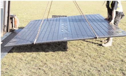
Before allowing traffic onto the ground protection plates, fully tighten each bolt using a 24mm socket. Periodically check each joiner for tightness and re-tighten if necessary.
